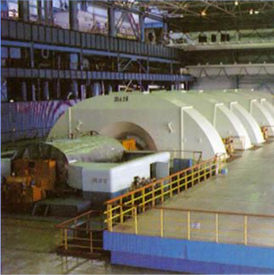
Turbogenerator 1000 Mwe, EJ Balakovo
